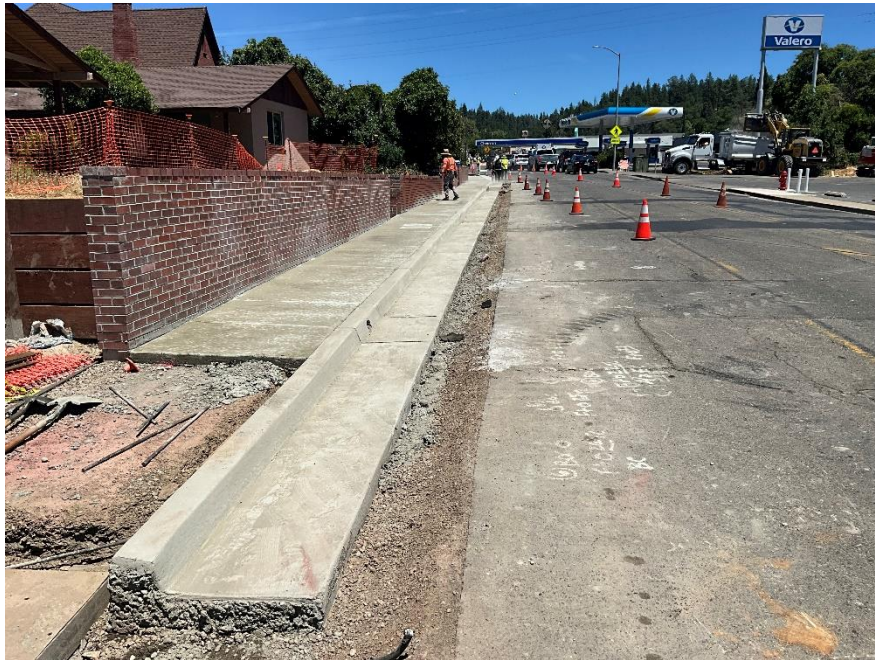
Retaining Wall Brick Cap (top), Sidewalk Finishing (bottom)
